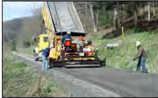
Paver-placement of TSA is preferred for longer sections of trail as pictured above.
